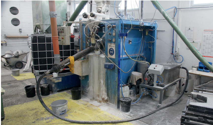
Fig. 1. A win-win situation: the mixing screws in this polymer concrete line are now purged with a specialty cleaning agent. This saves costs, protects employees and consumes only a small fraction of the chemicals used previously. © Färber & Schmid
